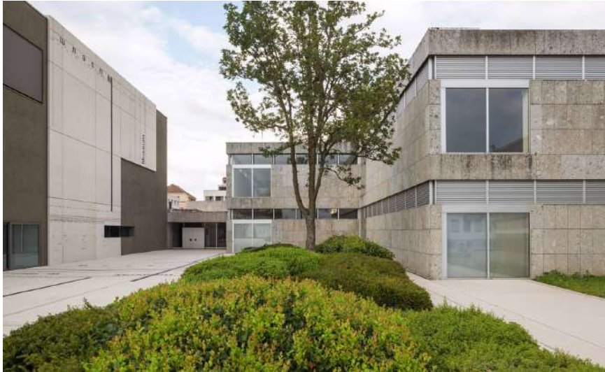
The project revolved around expanding the existing structure, which was originally designed by Hanns Schönecker and built between 1962 and 1974. Photography: Ulrich Schwarz, courtesy Kuehn Malvezzi
